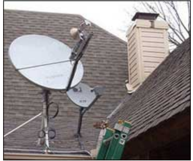
Satellite dish or receiver installed on a house. These dishes point to a geostationary satellite.
