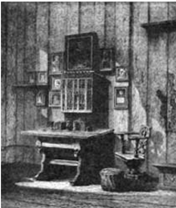
Saint Martin's study about 1850. On the right can be seen the ink stain and the broken plaster on the wall.
