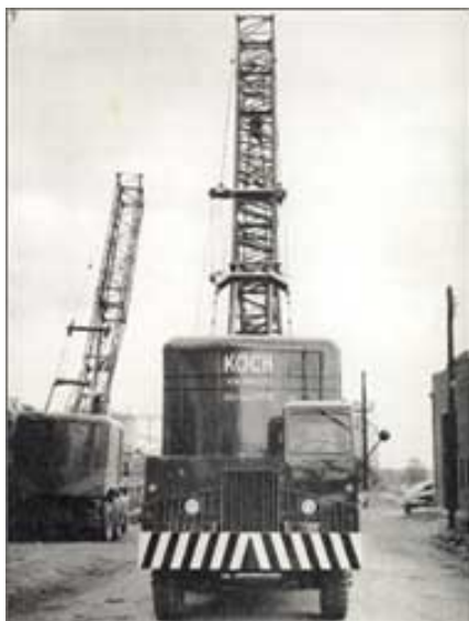
Karl Koch Erecting Co. built the Twin Towers.
