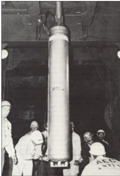
Nuclear explosive "Salmon" (5.3 kt) being lowered into its emplacement hole at Hattiesburg, Mississippi in 1964.
