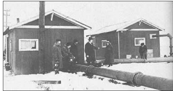
Ether-drift experiment conducted by Michelson in 1924.
