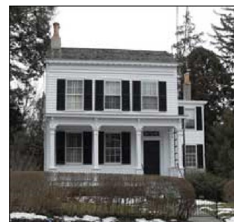
Einstein house in Princeton, New Jersey.
